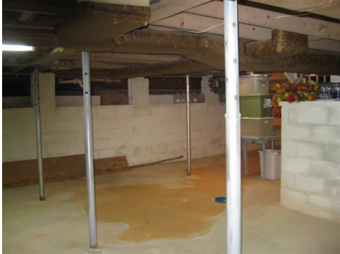
Basement Interior Access Only
